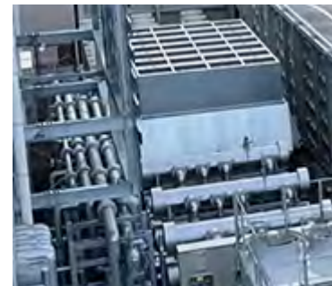
Chiller that improves energy efficiency by dividing the system into two temperature zones for different applications
