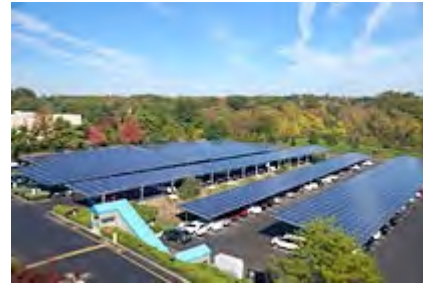
Photovoltaic panel installation in the company parking lot (United States)
